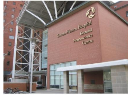
Toronto Western Hospital
